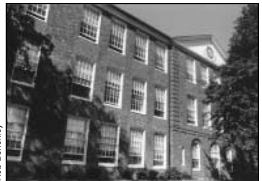
The Academy Hill School, built in 1928, has been adapted as apartments for senior citizens.
