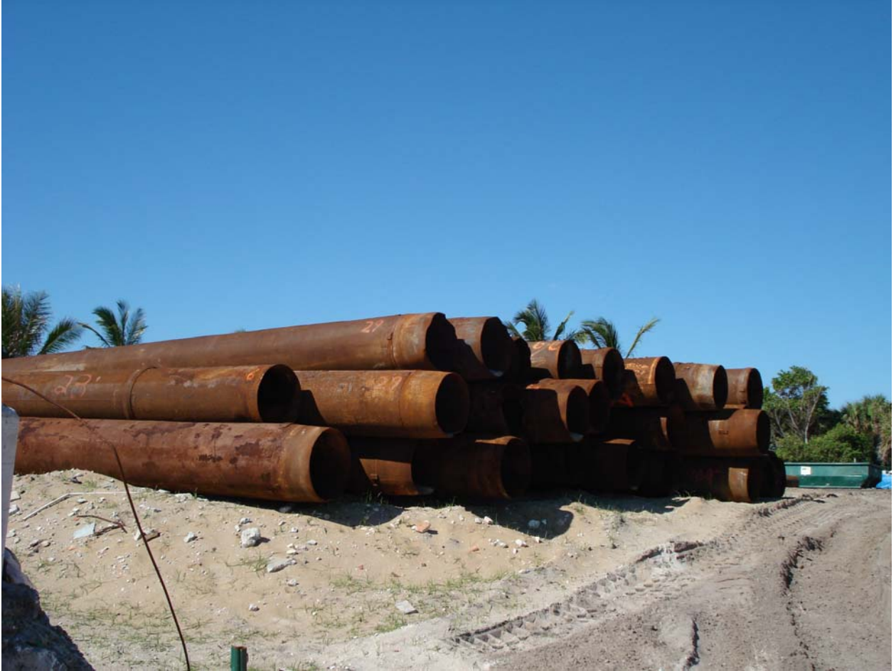
Figure 2. Close-up of Stockpiled Beach Pipe Sections. Pipe sections are typically 40 feet long by 30” diameter and are generally stockpiled in strategic locations for use on the beach. Typically 6 sections of pipe can be transported by flatbed truck and an end loader is required to move the pipe.
