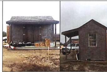
2. Existing Shed (Front/Side View)
