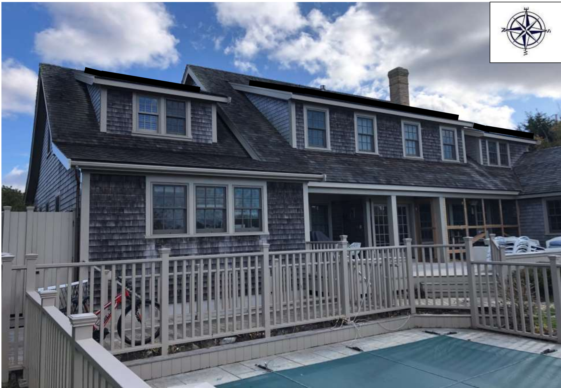
Rear Elevation (West Side)
