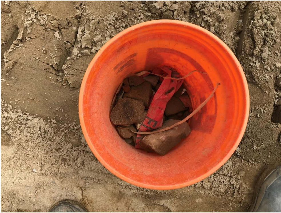
~ 1gl. small bricks, one red tape and few concrete blocks were collected during template grading at the delivery area.
