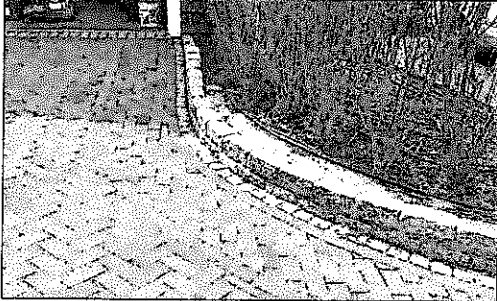
WOOD PLANKING REPLACED TO MATCH EXISTING COBBLE EDGING
