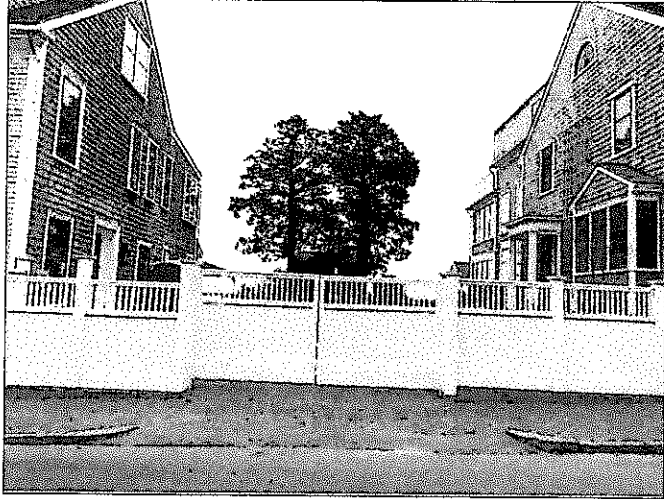
WOOD PLANKING REPLACED TO MATCH EXISTING COBBLE EDGING
