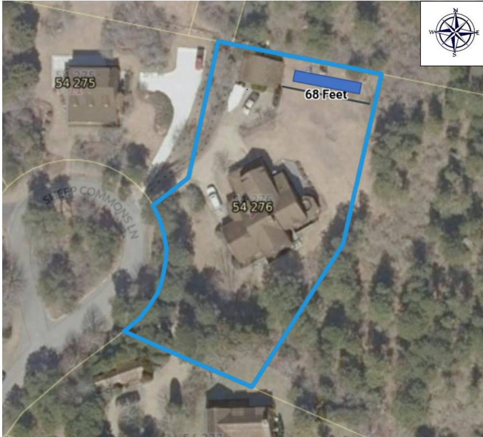
Google Earth image of showing ground mount solar array, not visible from the street
