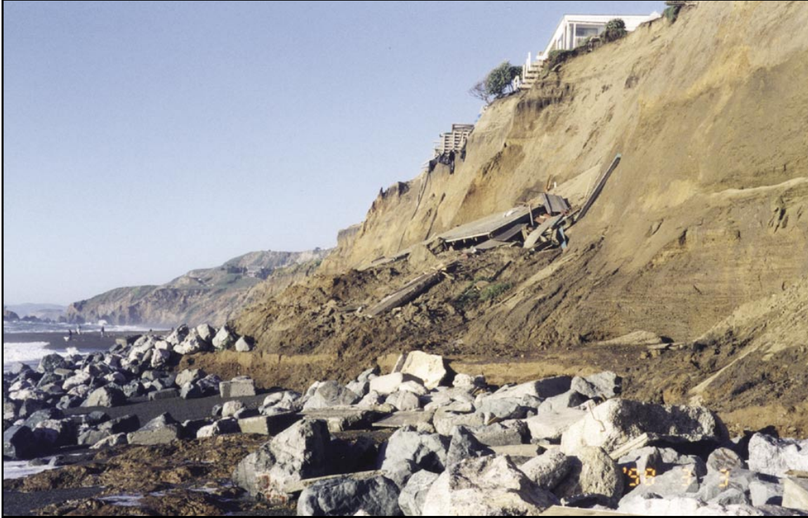
Figure 3. Remnants of previous rock revetment scattered across the beach after the 1998 El Niño event.
