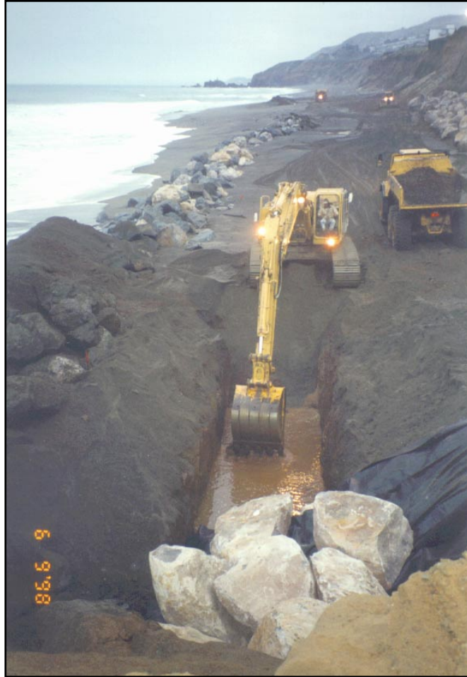
Figure 9. Keyway excavation below mean sea level required strategic construction timing with respect to tidal conditions.
