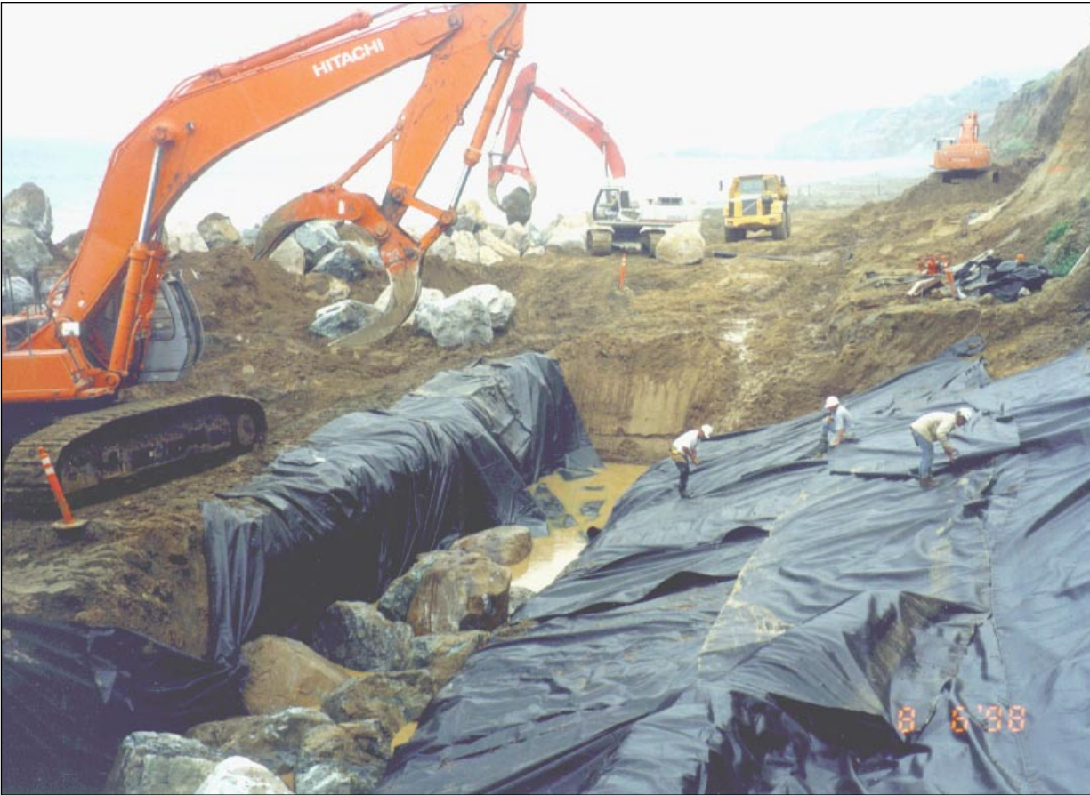
Figure 8. Filter fabric is being placed in the keyway and along the base of the revetment prior to stone placement.
