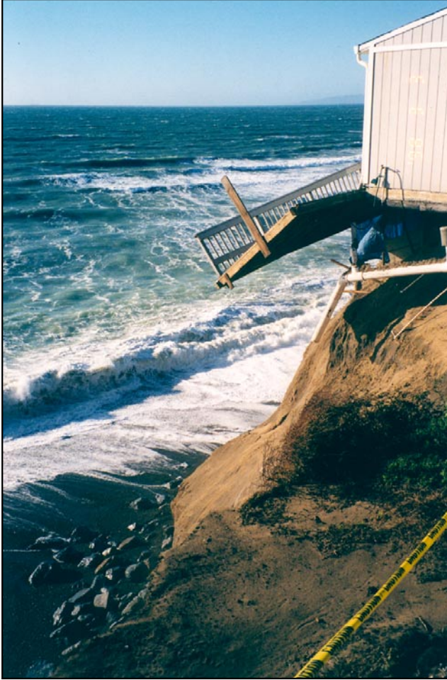
Figure 7. Offshore wave height may exceed 20 feet and wave surge from shore break attacks the base of coastal bluffs during high tides.
