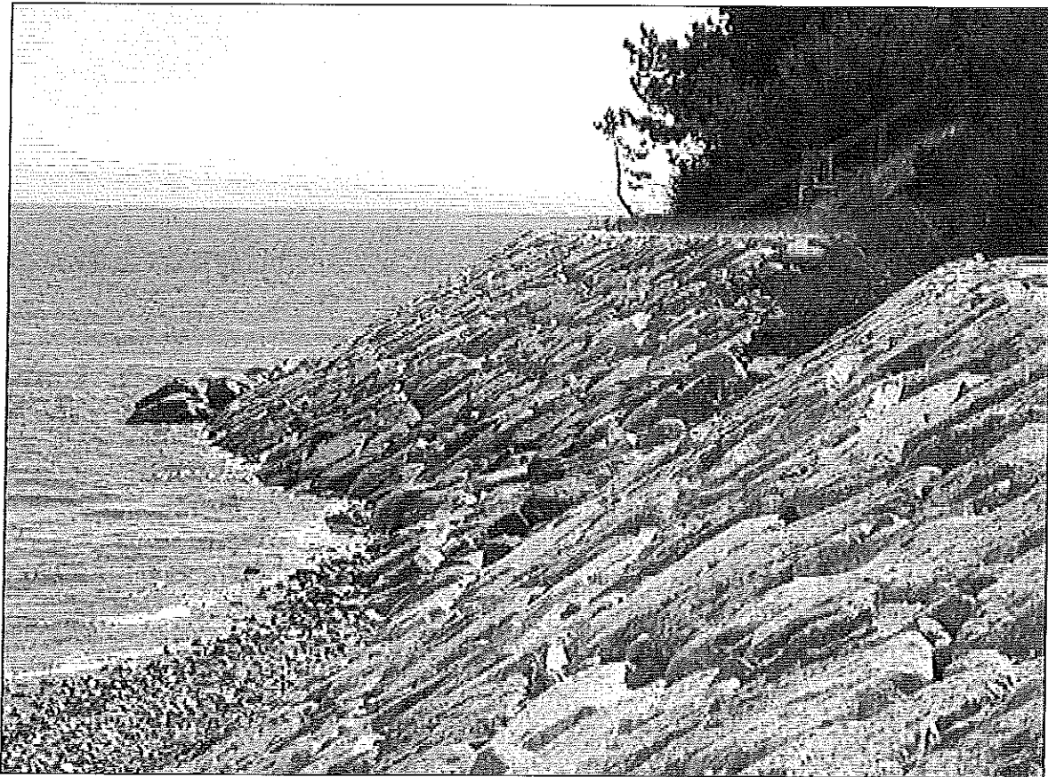
Figure 2: View of completed Triton Way revetment reconstruction that occurred during the 2006/2007 winter season ( source: Woods Hole Group, Inc. website ).
