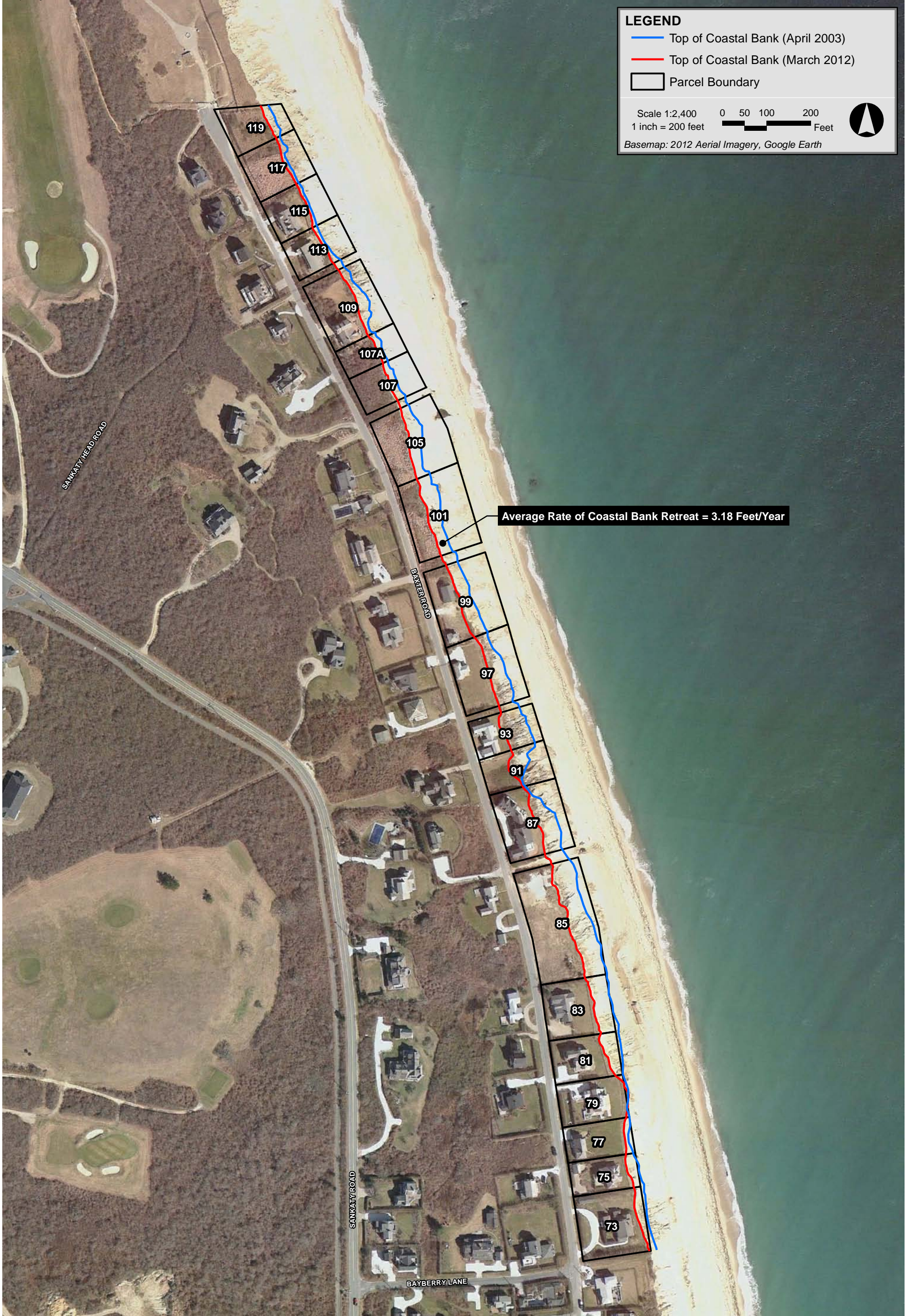
Baxter Road and Sconset Bluff Storm Damage Prevention Project Nantucket, MA
